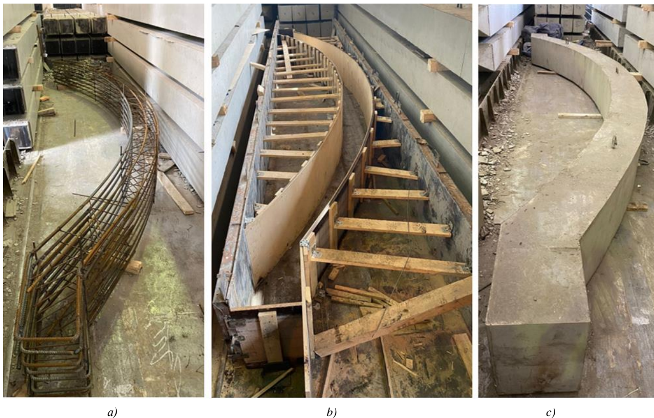
Fig. 3. Visualization of the process of creating a reinforced concrete structure: a — reinforcement carcass; b — single formwork; c — final arched beam on the edge
