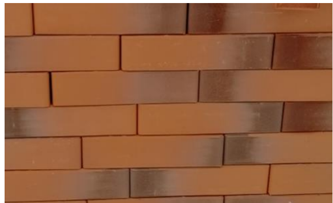
Fig. 7. Bavarian masonry using the engobated ceramic bricks (similar composition of K-2, K-3 + own brick color)
