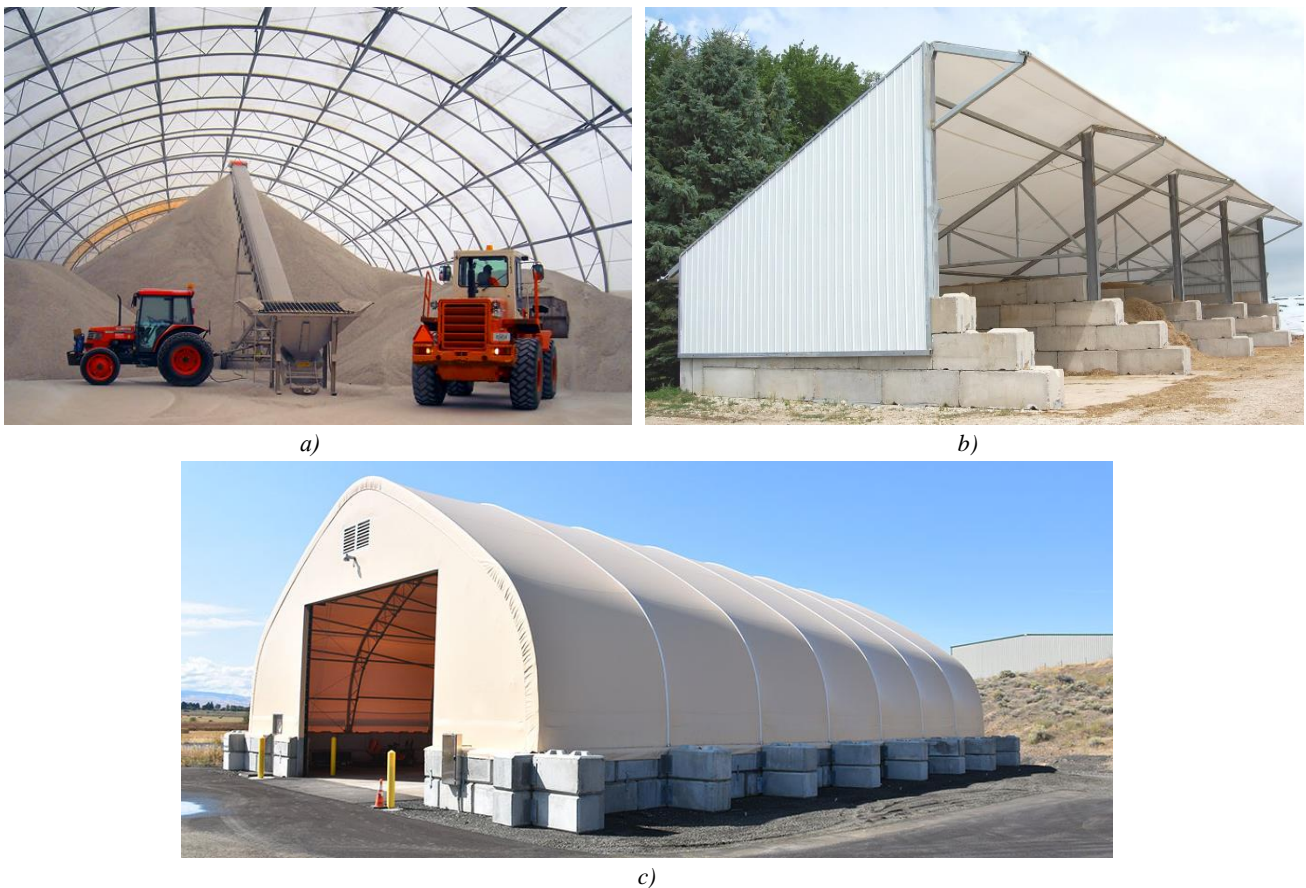
Fig. 2. Examples of typical buildings for the agro-industrial complex of Accu-Steel, USA: a – vaulted form made of metal frame and fabric covering with low side panels (Advantage series); b – with a gable roof made of metal frame, external and internal walls made of reinforced concrete blocks to accommodate an operational horizontal load (Crossover series); c – a parabolic-shaped frame made of metal trusses and low load-bearing walls made of reinforced concrete LEGO blocks with the same buttresses (Integrity series) [8]
