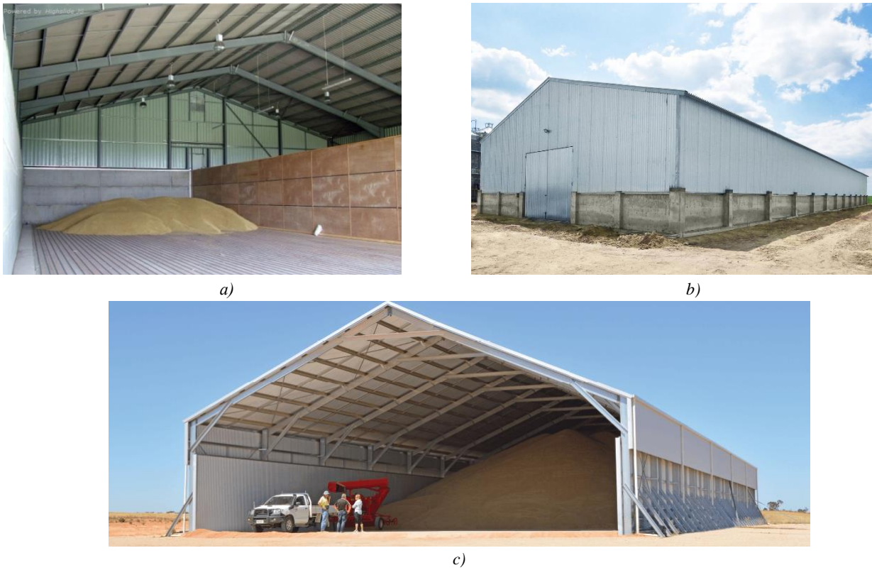
Fig. 1. Examples of domestic metal-framed structures of warehouses for storing agricultural products: a – with prefabricated inner walls accepting horizontal operational load; b – with external load-bearing reinforced concrete walls at the filling height; c – with wall panels, rod buttresses and additional connections
