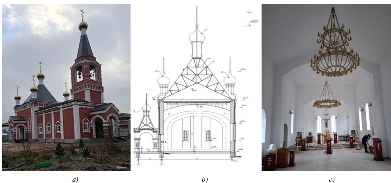
Fig. 1. Church of St. Tikhon, Patriarch of Moscow: a — exterior of the temple; b — section of the church considering account the built-in arched beam structure; c - view of the church towards the altar from the inside
