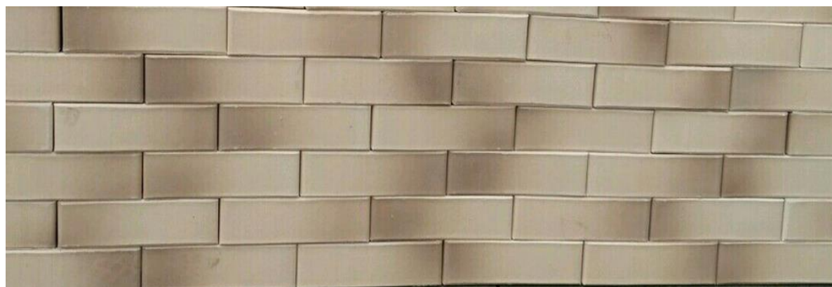
Fig. 9. Decorative bricklaying using the degrade effect (engobe compositions B-2, K-4)
