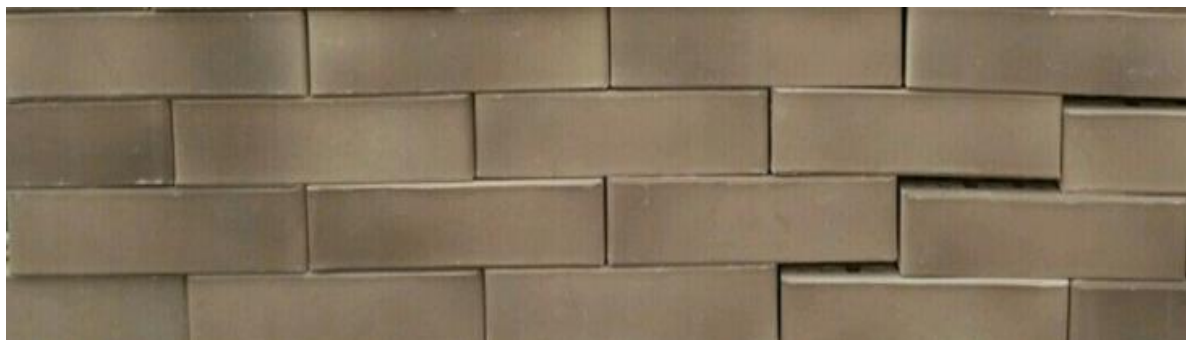
Fig. 8. Decorative bricklaying using the degrade effect (B-3, K-2, K-4 engobe compositions)
