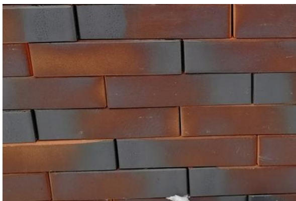
Fig. 6. Bavarian masonry using the engobated ceramic bricks (acid composition G-1, K-3 + the color of the baked brick)
