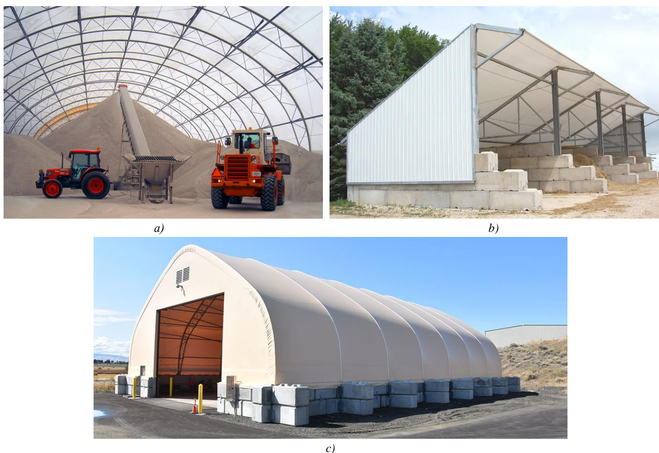
Fig. 2. Examples of typical buildings for the agro-industrial complex of Accu-Steel, USA: a – vaulted form made of metal frame and fabric covering with low side panels (Advantage series); b – with a gable roof made of metal frame, external and internal walls made of reinforced concrete blocks to accommodate an operational horizontal load (Crossover series); c – a parabolic-shaped frame made of metal trusses and low load-bearing walls made of reinforced concrete LEGO blocks with the same buttresses (Integrity series) [8]
