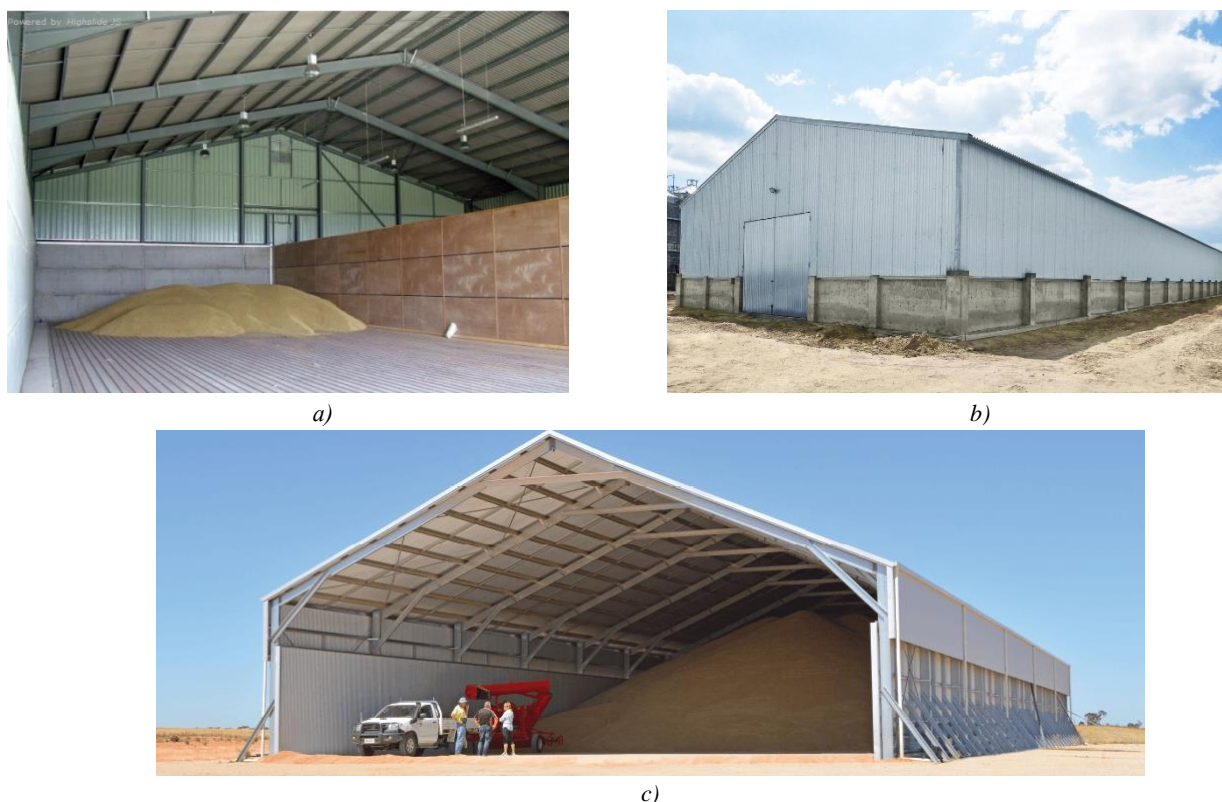
Fig. 1. Examples of domestic metal-framed structures of warehouses for storing agricultural products: a – with prefabricated inner walls accepting horizontal operational load; b – with external load-bearing reinforced concrete walls at the filling height; c – with wall panels, rod buttresses and additional connections
