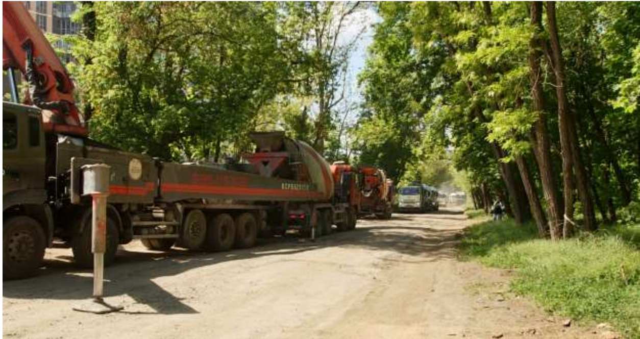
Fig. 5. Working site of CMT 2
