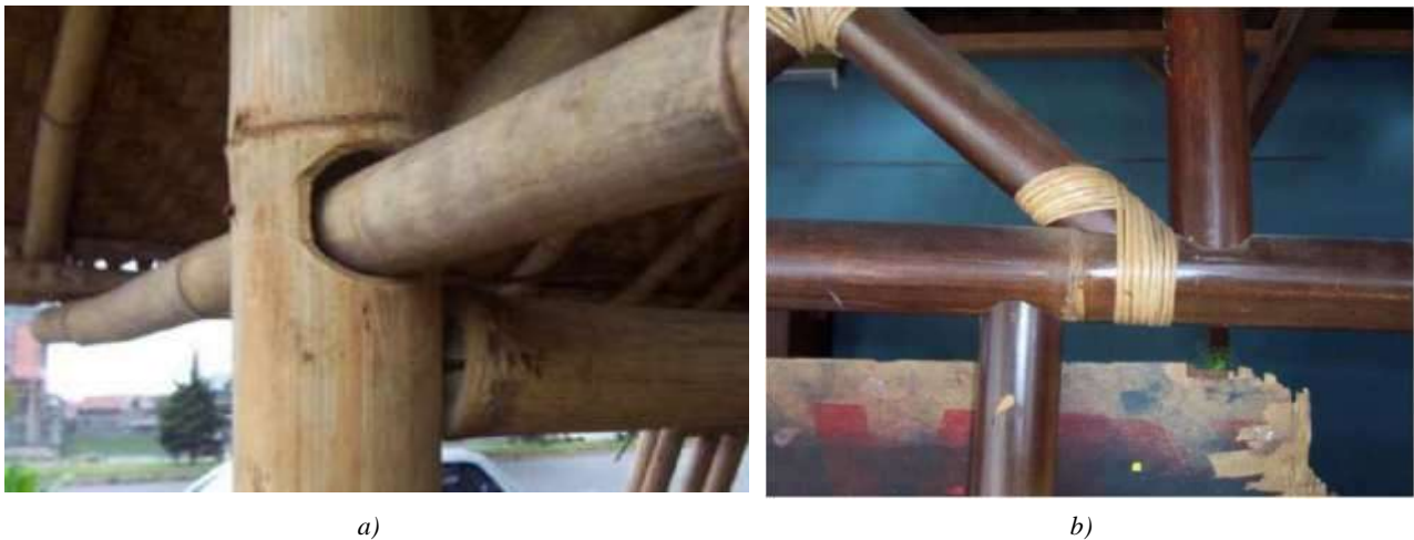
Fig. 1. Examples of connecting bamboo rods: a — through; b — strapping
